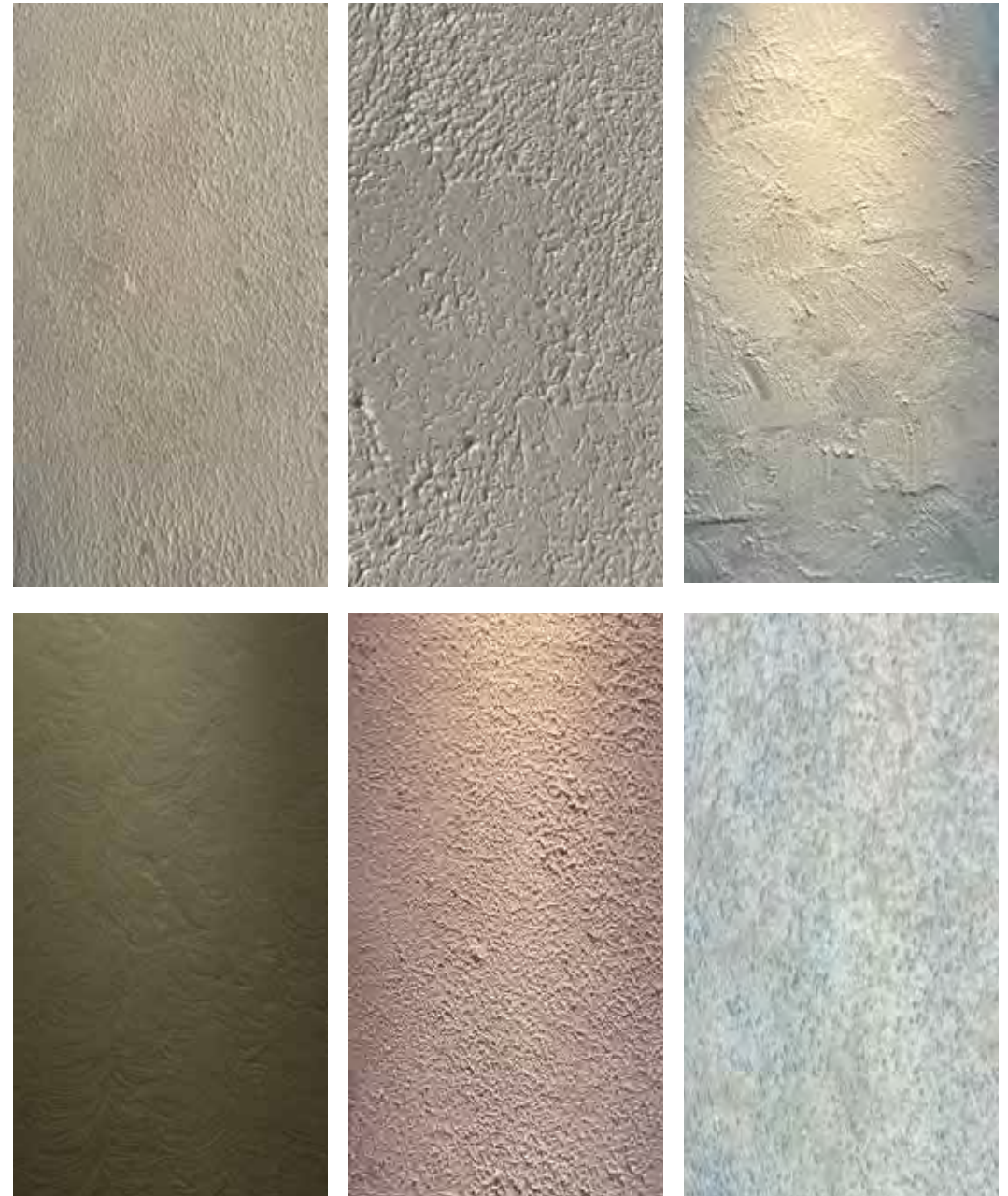
Figure 32: Textures by different applying techniques together with color. Depending on how the different parameters are, complexity and coherence differ. The light also are a factor that turns the texture on and off as well as reducing or articulating.
